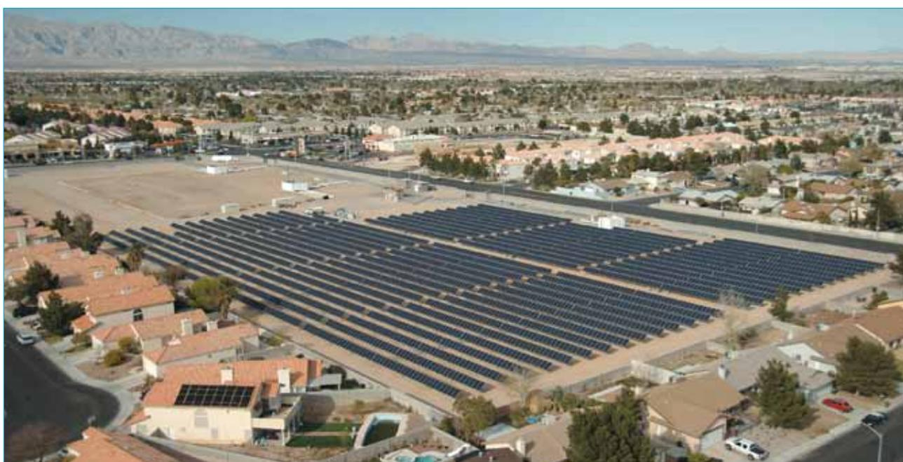
Figure 2. Horizontal single-axis trackers optimized for space-constrained sites.
