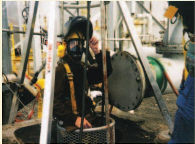
At a Florida industrial site, a welder puts on safety gear before descending into a well to make repairs. A downhole survey had been used to pinpoint a hole in the well casing.
