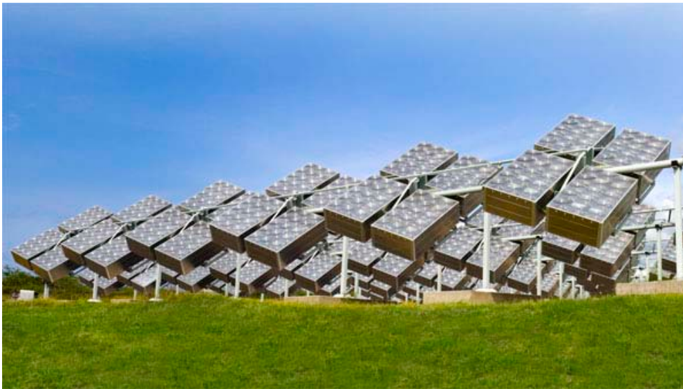
Maui, Hawaii – Gen3 CPV Installation
