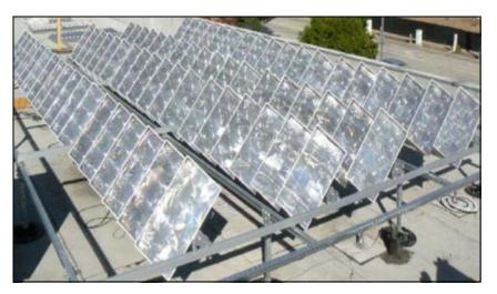
Rooftop CPV System – 350W panels for nonpenetrating roof installs
