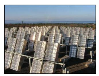
Gen-III CPV System – 16.2 kW Ground Mount System w/ 36 Gen III modules
