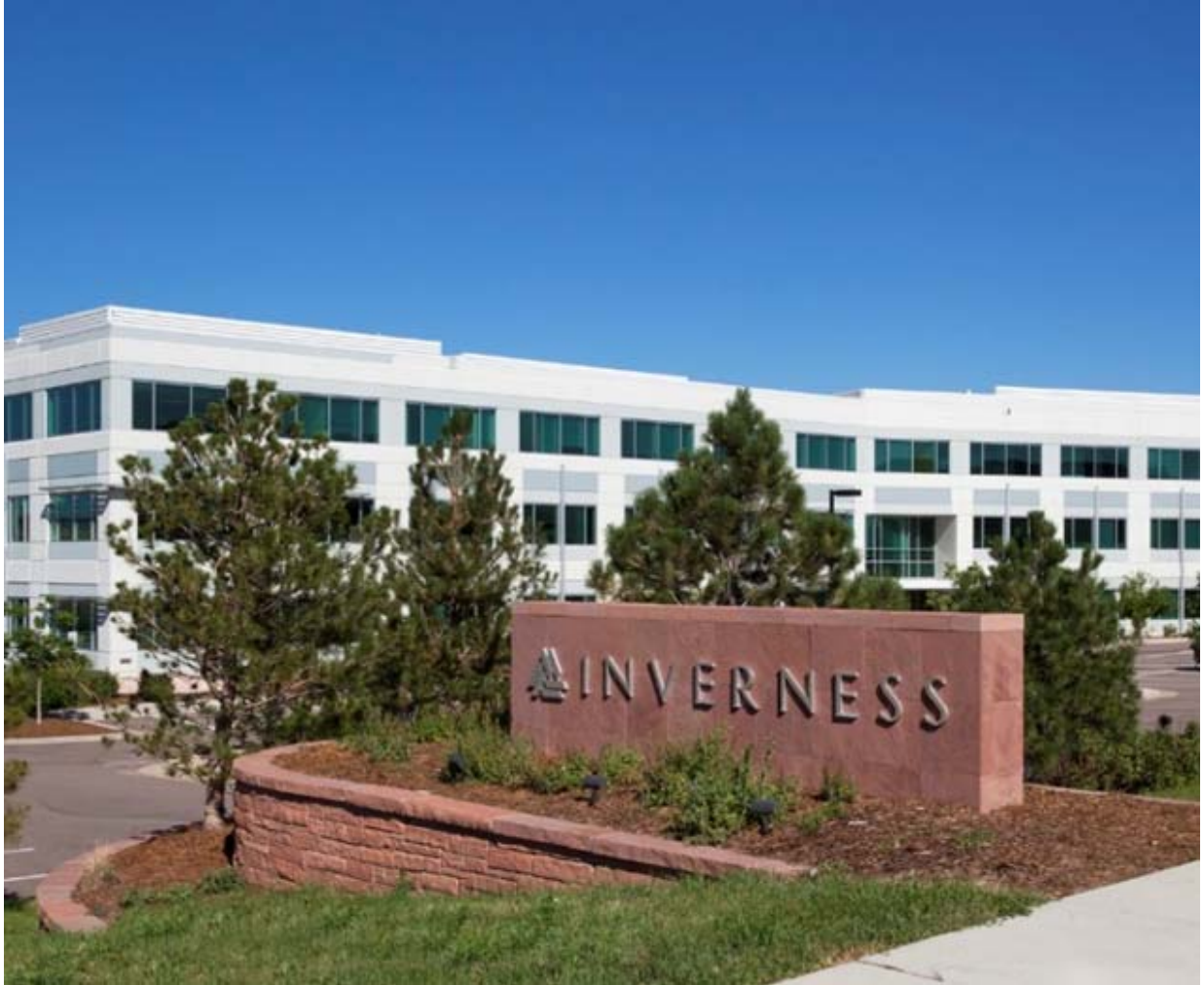
One of the Company's properties, located in Denver, CO.
