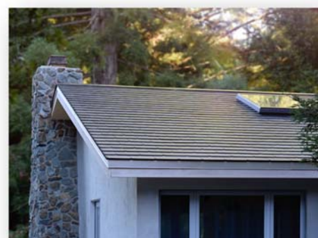
First Solar Roof Installations Completed
