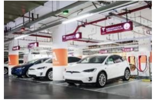
50-Stall Supercharger Station in Shanghai
