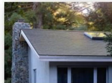
First Solar Roof Installations Completed
