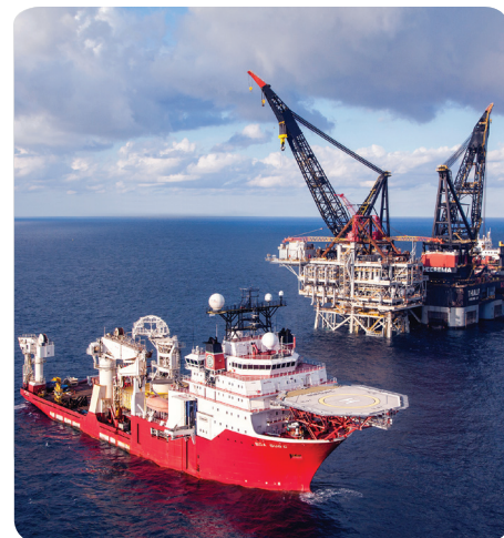
Tamar platform installation Photo courtesy of Albatross Aerial Photography Ltd.
